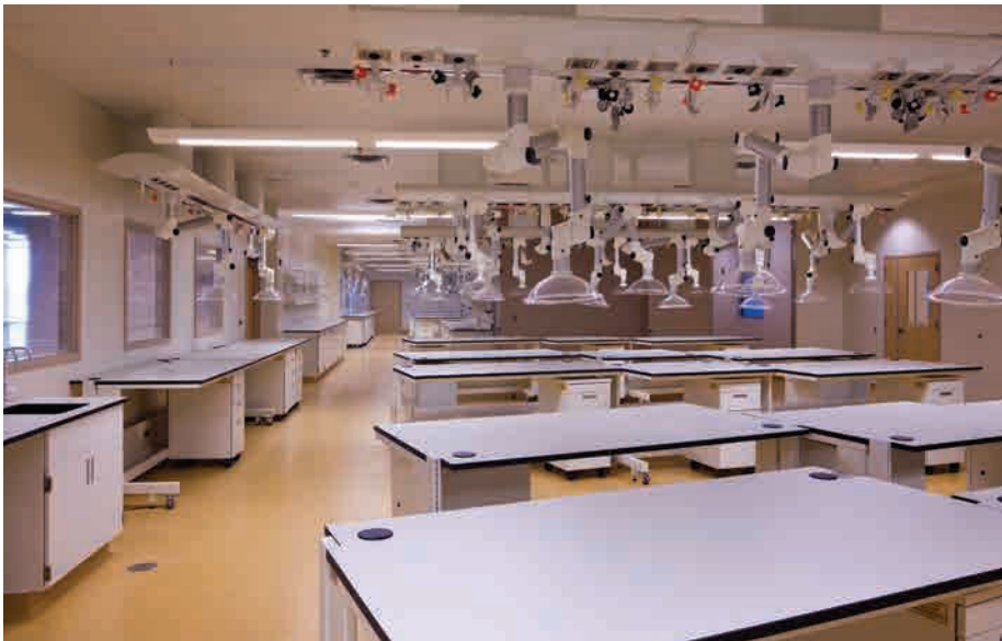
Left, Bottom Left and Bottom Right: Many labs feature direct/indirect lighting and extensive use of occupancy sensors with manual override
